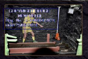
Roof and floor convergence issues are quite frequent inside the downcast Coal Mine. Taking preemptive measures to tackle such incidences, therefore, is one of the major challenges on the part of the mining professionals over the year.
